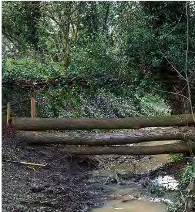
Figure 10: Evidence to action case study of leaky dams in Essex. Images from Floods Team at ECC.
