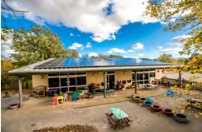
Figure 8. Solar panel on the roof of Danbury Park Community Primary School
